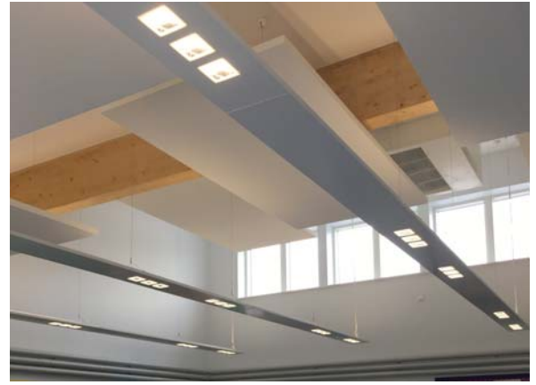
▲ Acoustic ceiling panels, Houghton School.
